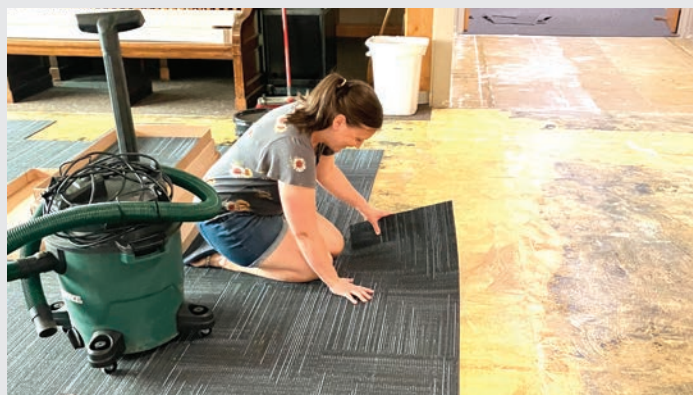
Sarah (Butterfield) Diaz installs a carpet square in the school chapel.
